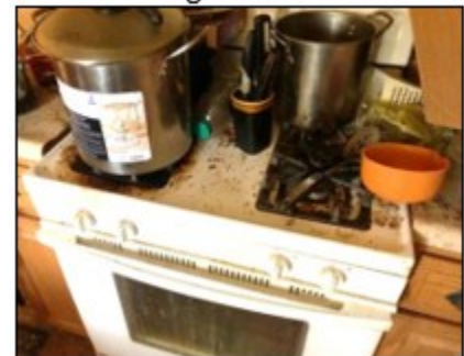
Figure 20. Combustible Items on Gas Range
